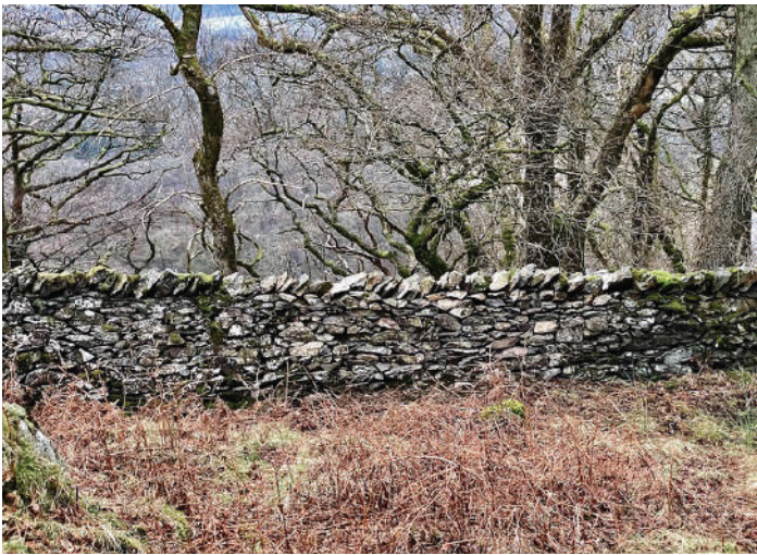
1. A repaired section of wall, which is up to 25% air
