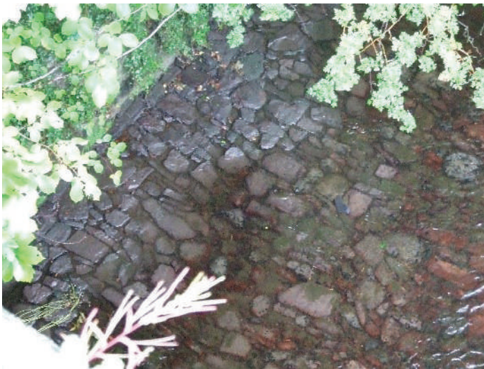
Fig.5 - Protective stone layer to bed of river
