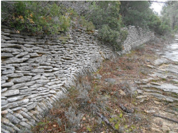
Fig.3 - Diagonal bottom course, Var France
